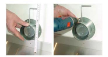
Fix the connecting piece to the wall using the screws and raw plugs provided.
